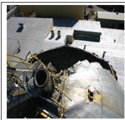
Source: CSB website - Views of the storage tank involved in the 2008 explosion at Packaging Corporation of America.
